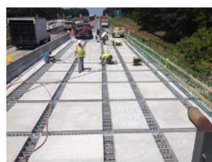
Precast Bridge Deck Connections
