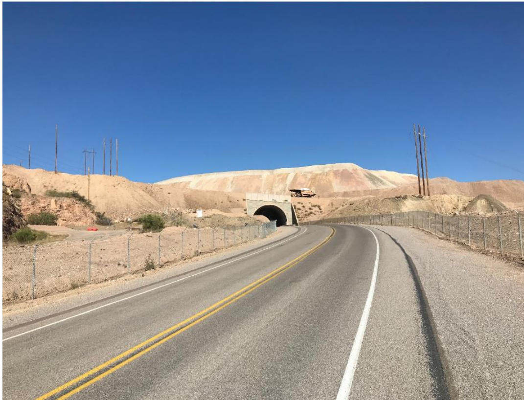
Public access highway below the arch
