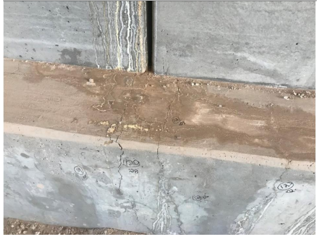
Vertical cracking
